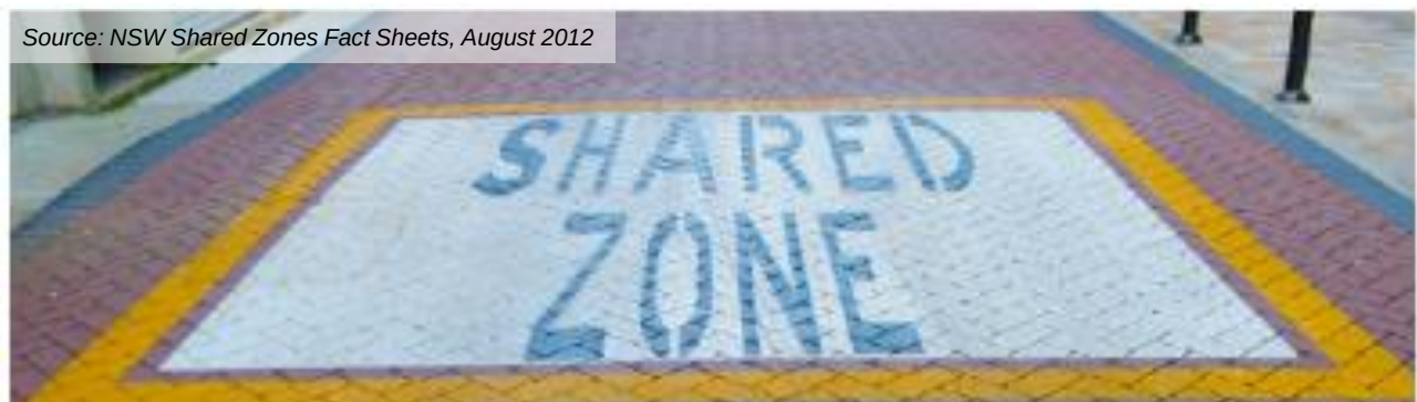
Figure 3.8 Shared Zone Raised Threshold Example
